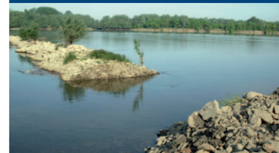
5 Reconstruction of groynes for revitalisation of Danube Island
