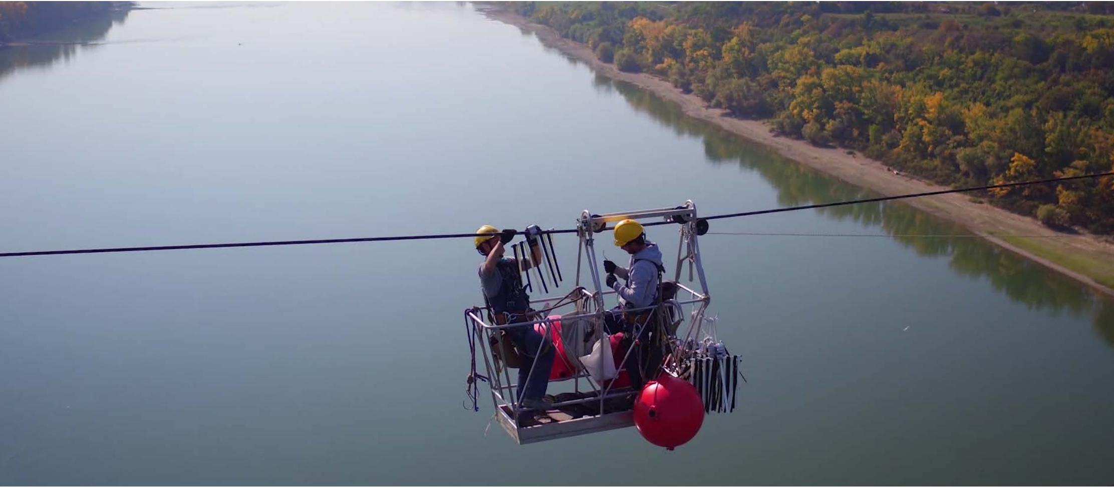
Close cooperation with the electricity providers: Marking of a high-risk power line crossing the Danube in Hungary.
